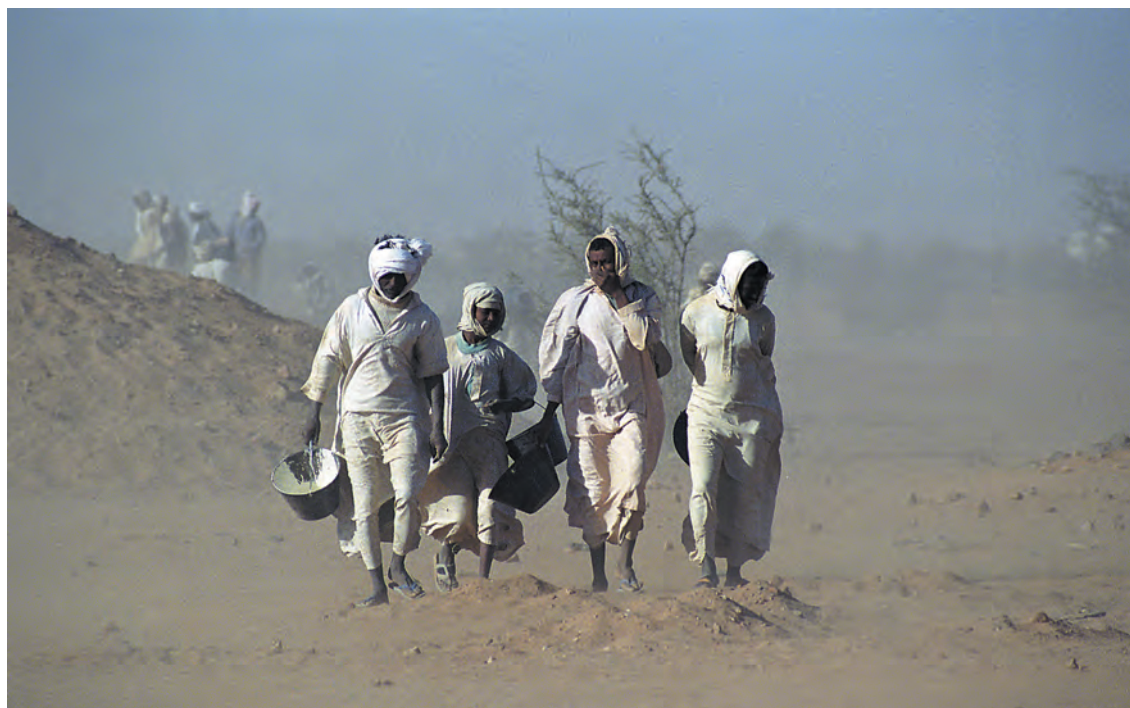
El Awlib, Meroitic temple complex, work in progress on site
